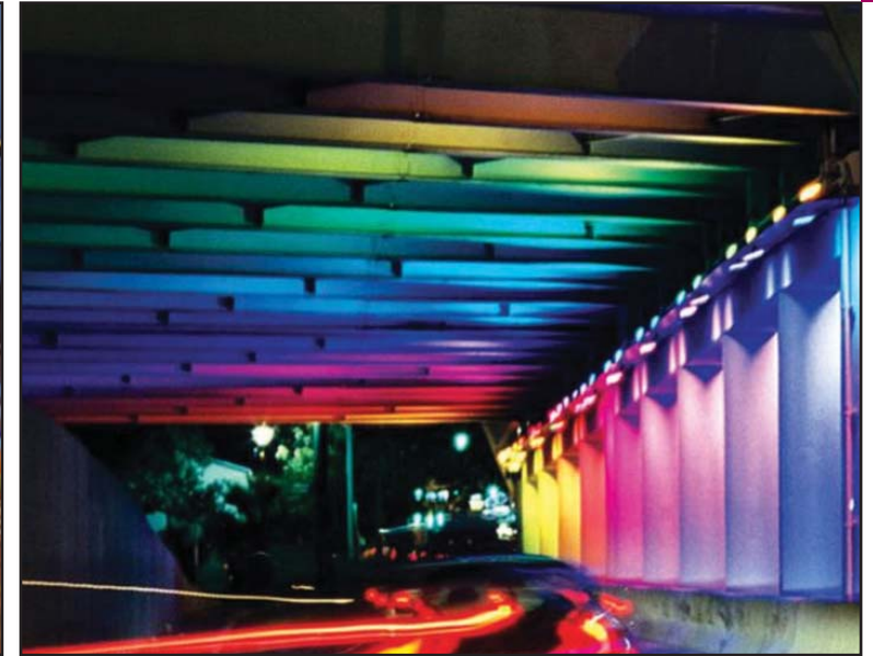
GATEWAY WITH COLORFUL LIGHT PATTERN ON RETAINING WALLS Bill FitzGibbon's Technicolor Underpass Installation | Beautifuldecay.com P. Russ Crest, 25 Oct. 2012, Web. 26 Nov. 2015.
