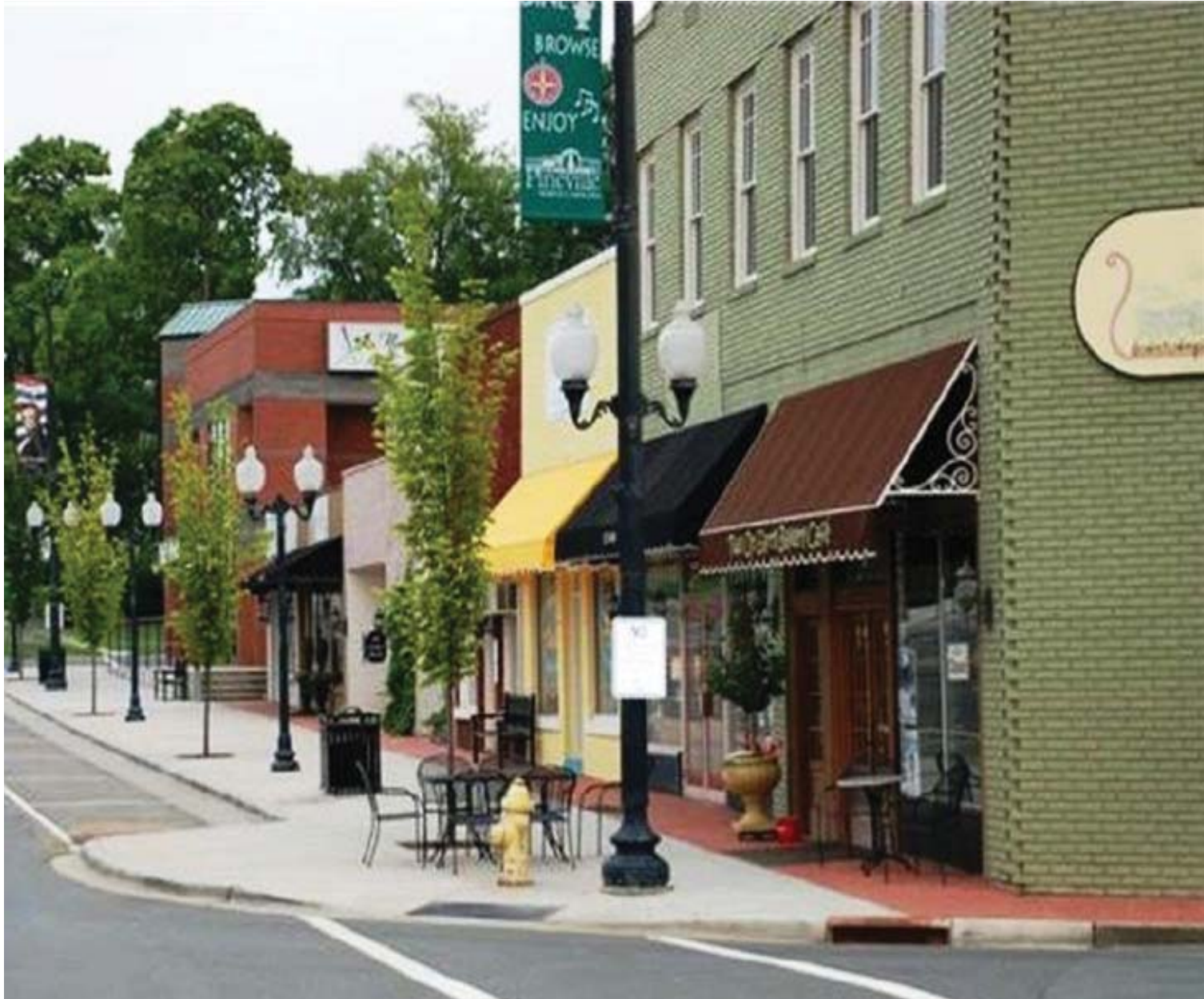
REPLACING OVERHEAD CABLES WITH VISUALLY PLEASING STREET LIGHTS Pineville, North Carolina | tourfactory.com , Web. 30 Nov. 2015.
