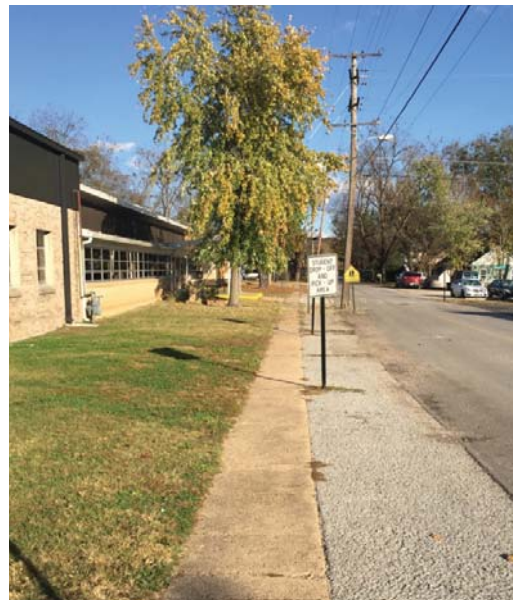
POOR ROADSIDE FRONTAGE ALONG SCHOOL ROAD
