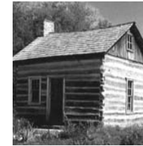
First McDonald County Courthouse 1849-1857
