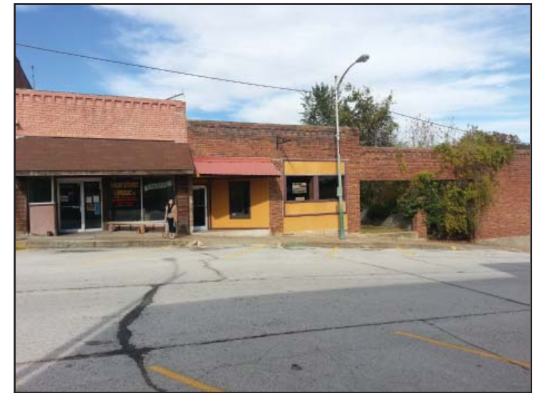
View to the north on Main Street looking at brickwork and overgrown plant growth
