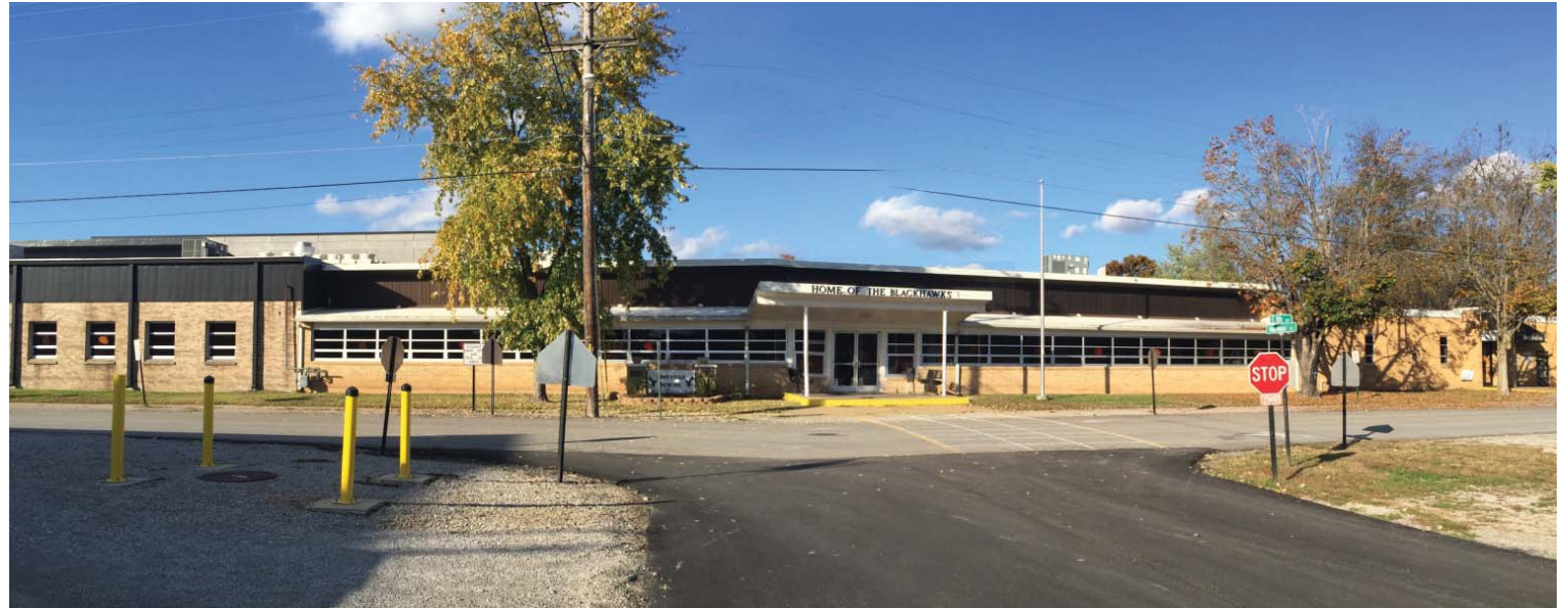
NON EXISTENT SIDEWALKS ALONG SCHOOL ROAD
