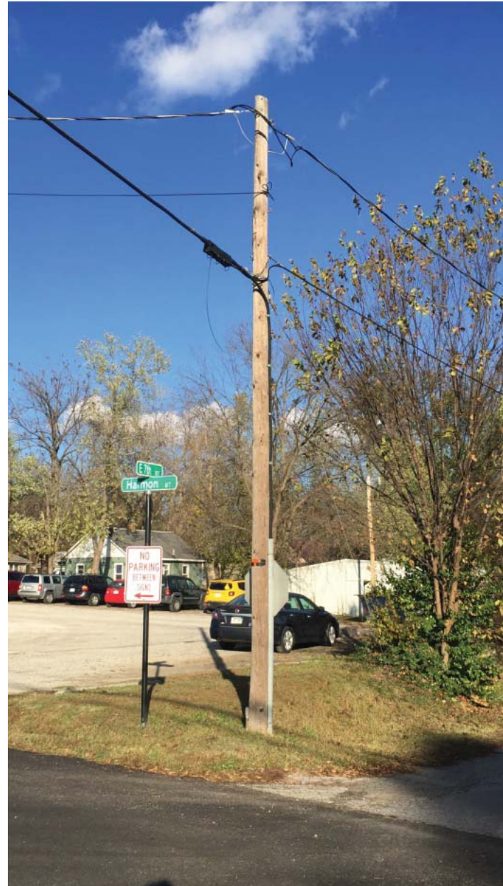
EXISTING OVERHEAD TELEPHONE LINES
