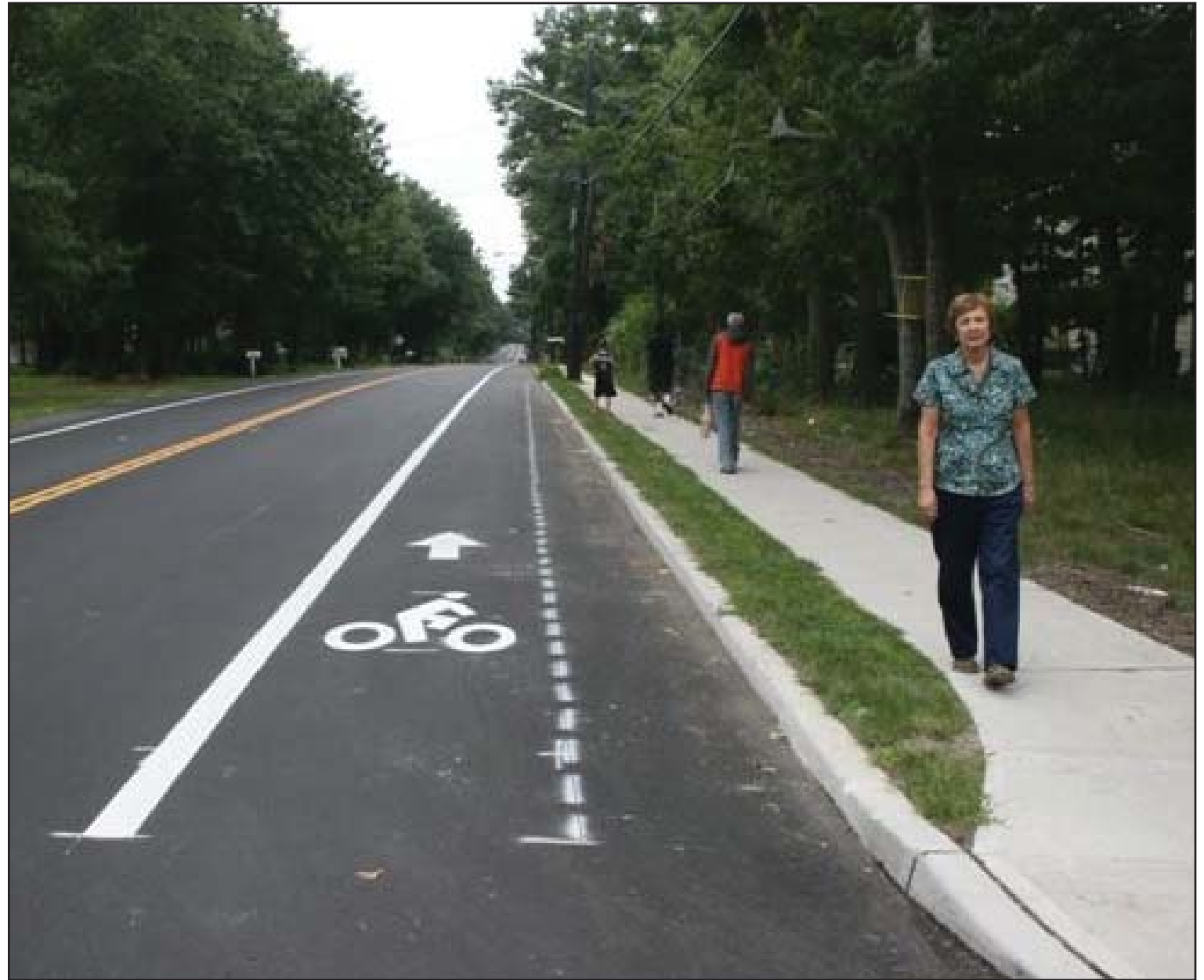
Stock image of a multi-use roadway which includes vehicular, bicycle, and pedestrian lanes. Tri-State Transportation Campaign. "Complete Streets." N.p., 2011. Web. 30 Oct. 2015. < http://blog.tstc.org/wp-content/uploads/2013/09/bike-lane-sidewalk.jpg >
