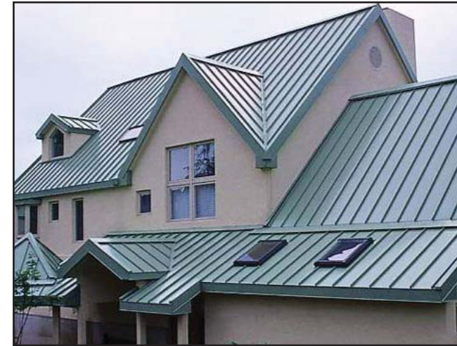
Standing Seam Metal Roof (Source: Yellow Hammer Roofing, Image by Yellow Hammer Roofing Inc.)
