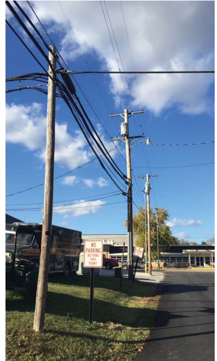
EXISTING OVERHEAD ELECTRICITY LINES
