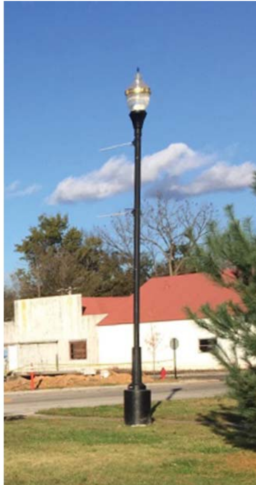
EXISTING STREET LIGHTS
