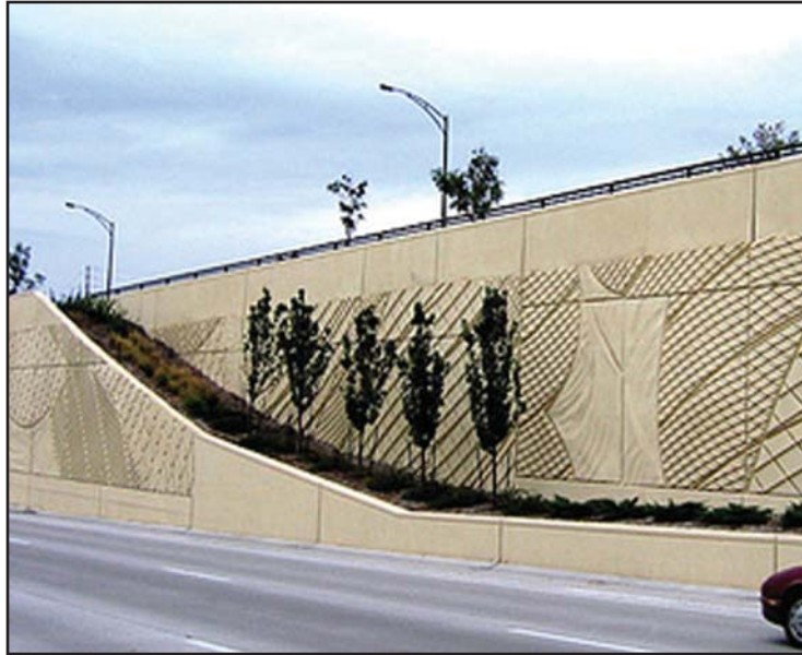
GATEWAY WITH RELIEF PATTERN ON RETAINING WALLS Kellogg/Woodlawn Interchange- Wichita, KS | flickr.com, P. Creative Design Res. 7 Apr. 2009, Web. 27 Nov. 2015.
