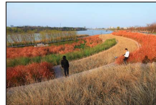
Elevated banks with vegetation made to control high flood waters
