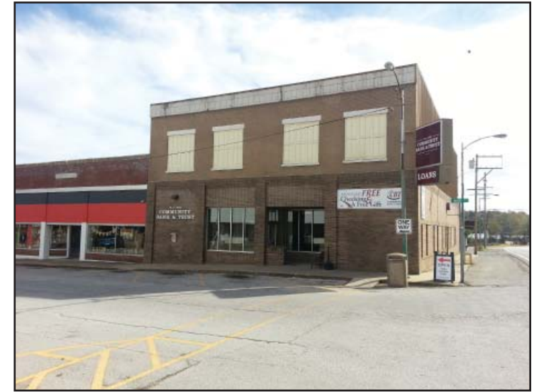
Community Bank and Trust facade
