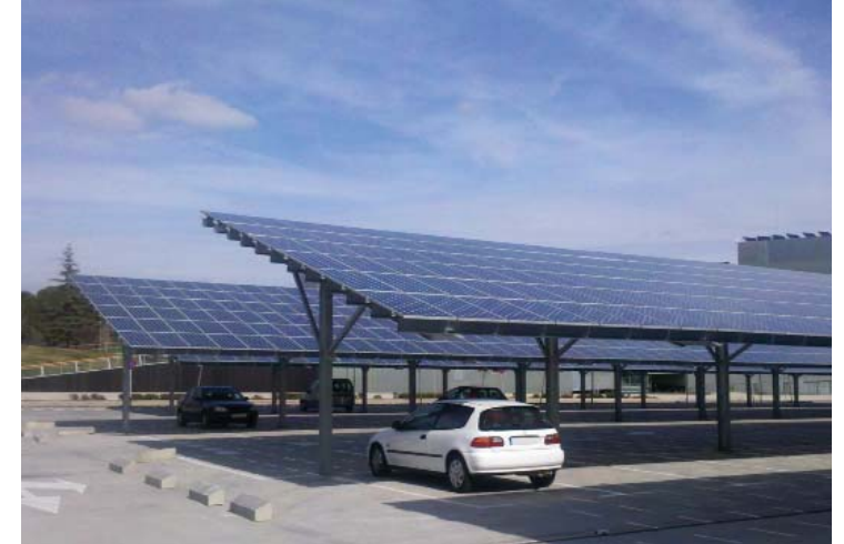
Solar Canopy (Source: Green Energy; Image by Unknown)
