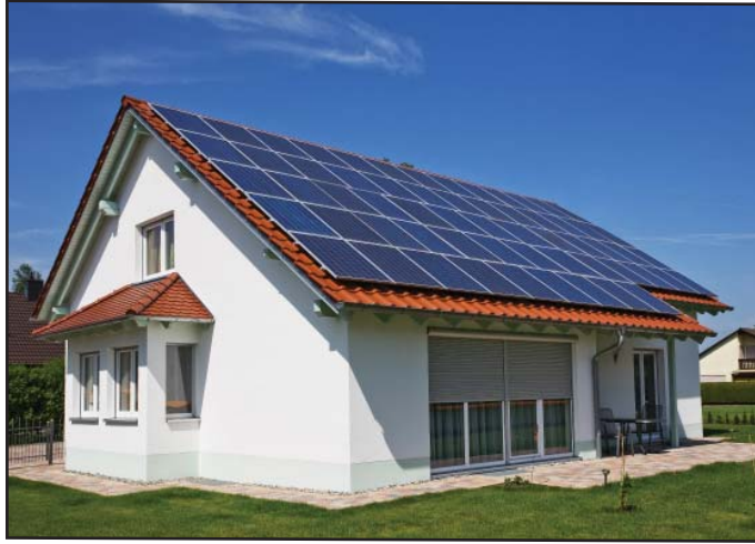
Rooftop Solar Panels (Source: Scitel Systems; Image by Unknown)
