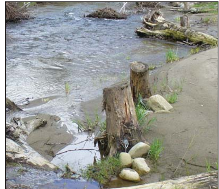
Installed large woody debris captures sediments.
